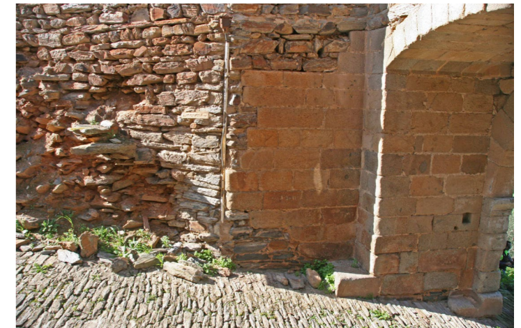
"Porta de Évora" Previous to project. 2016 © PP
